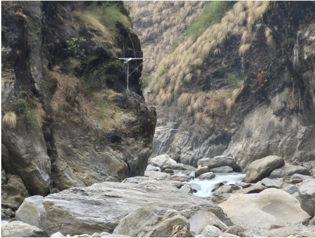
Figure 7-18: AWLR station installed just upstream of Balephi-Nyasim Confluence
