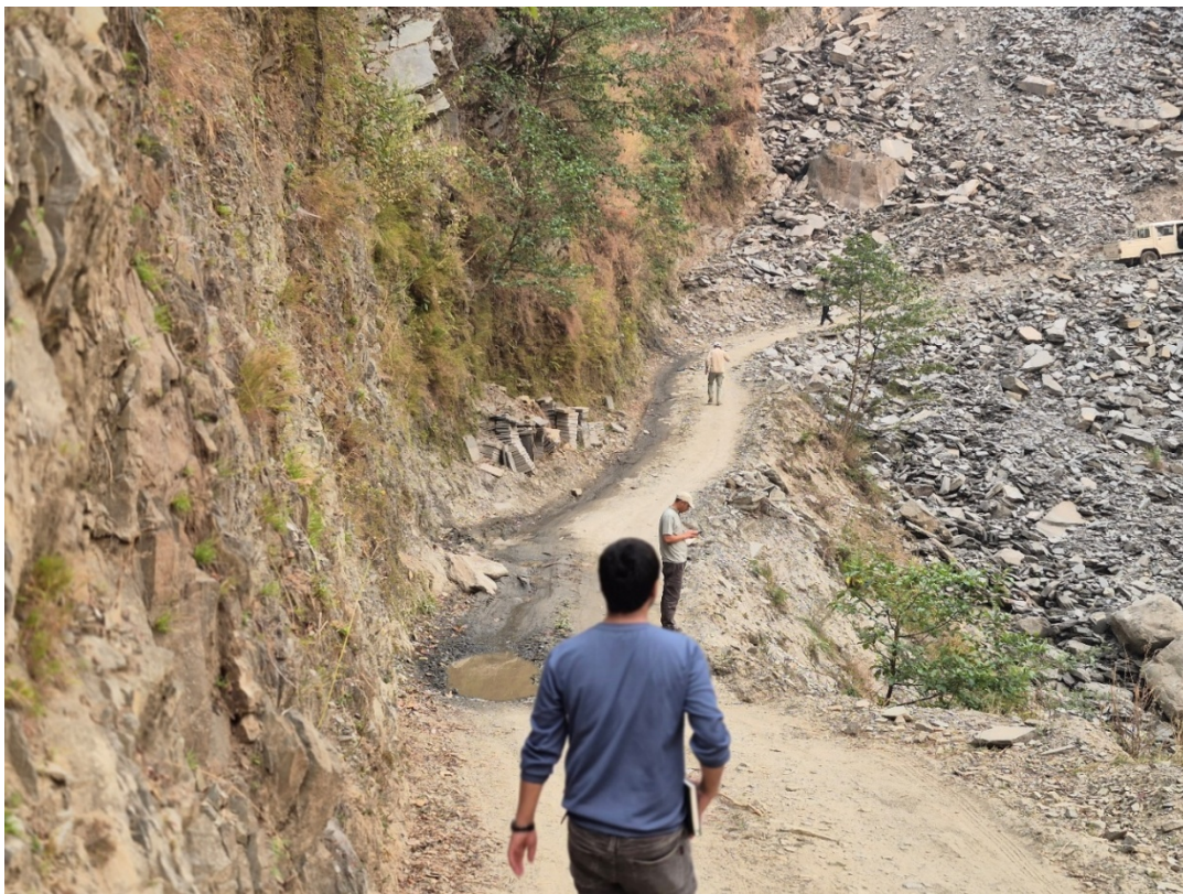
Figure 7-17 Road condition near Powerhouse
